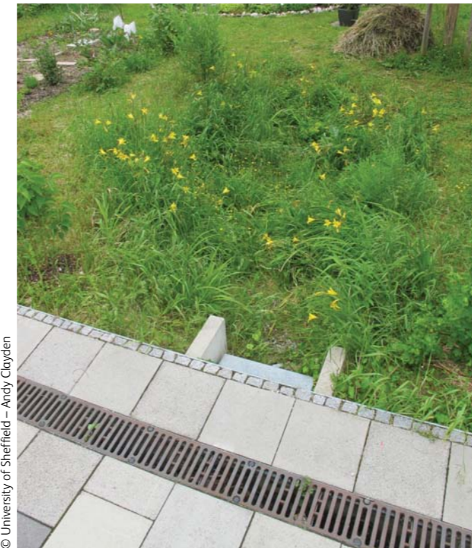
Figure 7.7: A swale is used to gather surface water from the residential area, and allow it to percolate slowly into the main drainage system. This reduction in the rate of surface water run-off allows the main drain systems to better cope with intense rainfall events.
