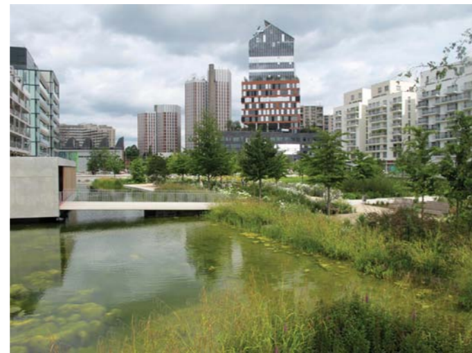
Figure 7.5: Retention pond in Billencourt, Paris.
