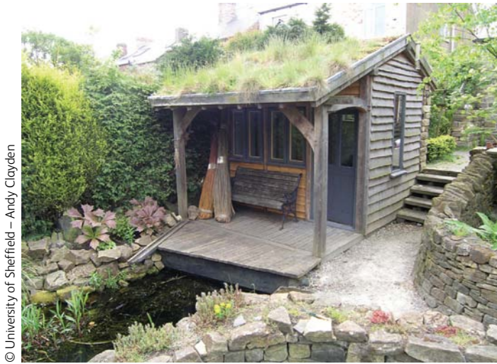
Figure 7.12: Garden building incorporates a veranda, providing an outdoor work or seating space in wet weather. The building is also used to manage rain water which is fed directly into the adjacent pond.
