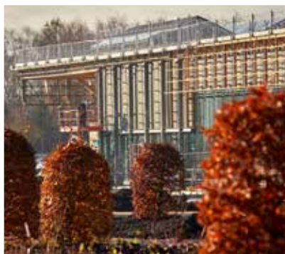
Left: The new Welcome Building at Bridgewater nears completion.
