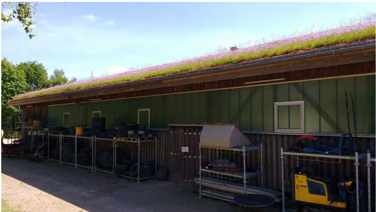
Figure 27 Machinery shed with green roof, Lorenz von Ehrens Nursery
