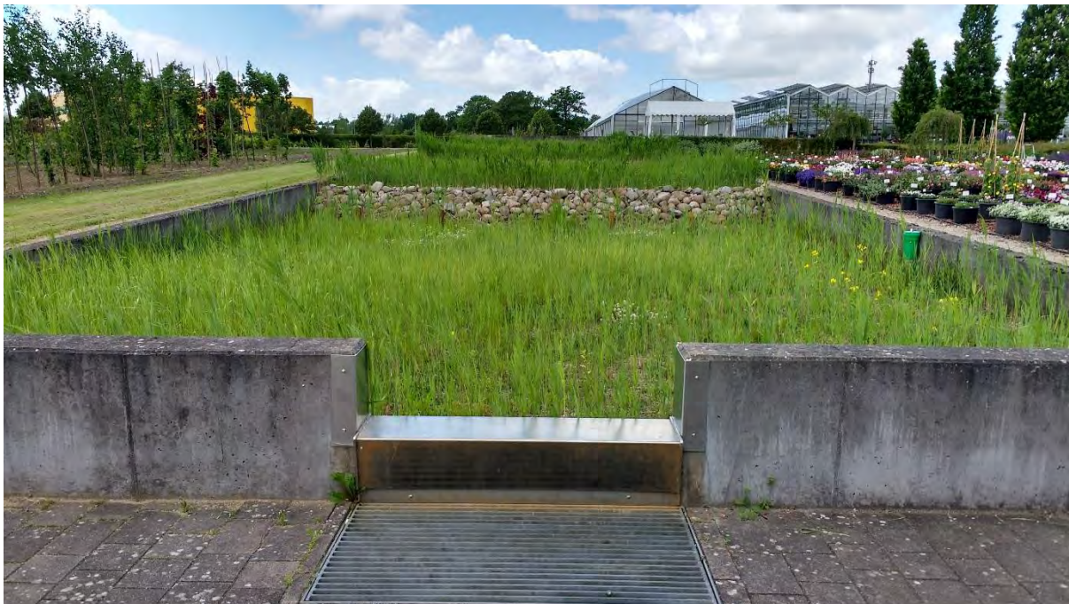
Figure 17 Sandbed filtration system, Centre of Horticulture, Ellerhoop
