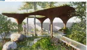
*palustris* and *Hesperaloe parviflora*. The pavilion is made of a steel subframe, clad with overlapping weathering steel sheets, giving it an organic and fluid form. Rainfall is harvested from the structure, filtering and slowing down its dispersal into the landscape.
